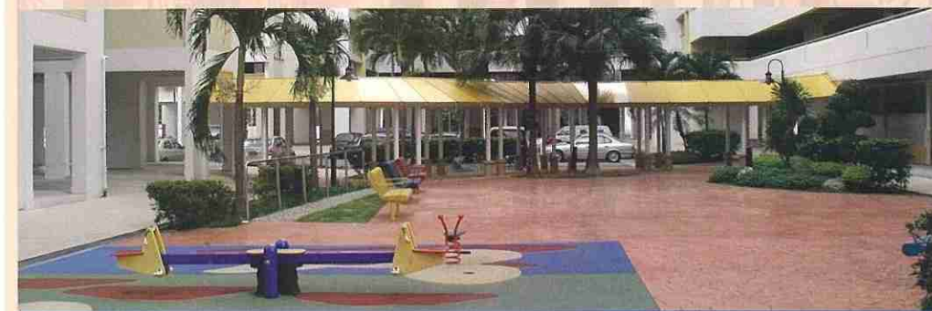
Covered Linkway at Blk 58 Dakota Crescent ( Completed in 2002 )
