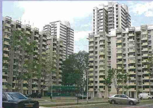
MUP at Blk 1 - 8 Marine Terrace ( Completed in 2006 )
