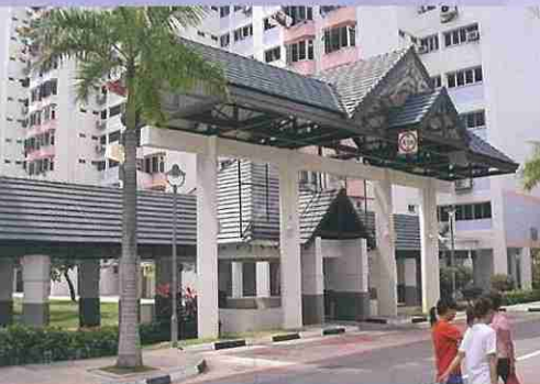
Drop-off Point at Blk 60/61 Marine Drive ( Completed in 2005 )
