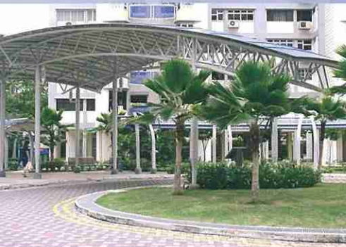
MUP at Blk 12 - 20 Marine Terrace ( Completed in 2004 )
