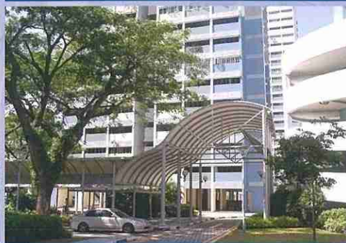
MUP at Blk 27 - 35 Marine Crescent ( Completed in 2002 )
