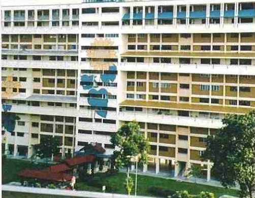
R & R at Blk 101 - 108 Serangoon North Ave 1 ( Completed in 2003 )
