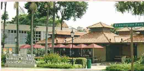
HUP at Chomp Chomp Food Centre ( Completed in 2004 )
